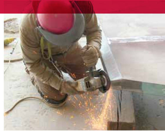
Grinding on a platform for weld preparation.
